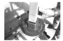
6. Repeat steps 4 & 5 with the other end of the tubing and the top op-nut. After the extension is assembled, allow it time to set-up. This time may vary with the type of adhesive used. Make sure that the op-nut ends will not slide off when lowering the extension into the valve can.
